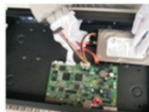
2. HDD data line and power line connection
